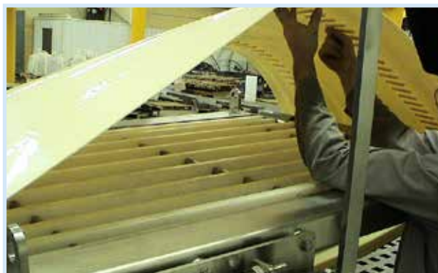
Belt repaired on site.
