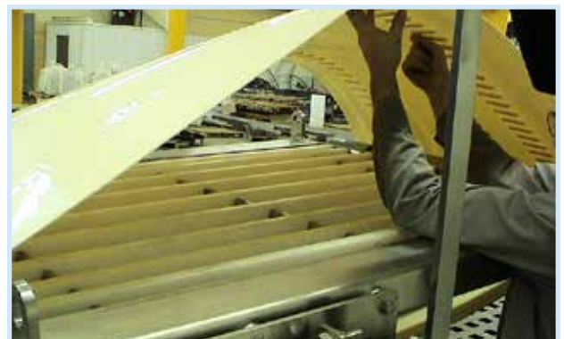
Belt repaired on site.
